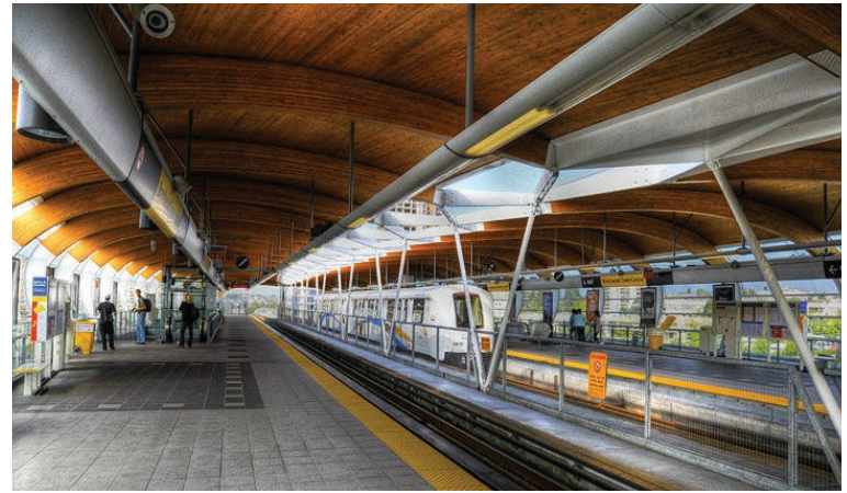
FIGURE 51 - BRENTWOOD SKYTRAIN STATION - PLATFORM
