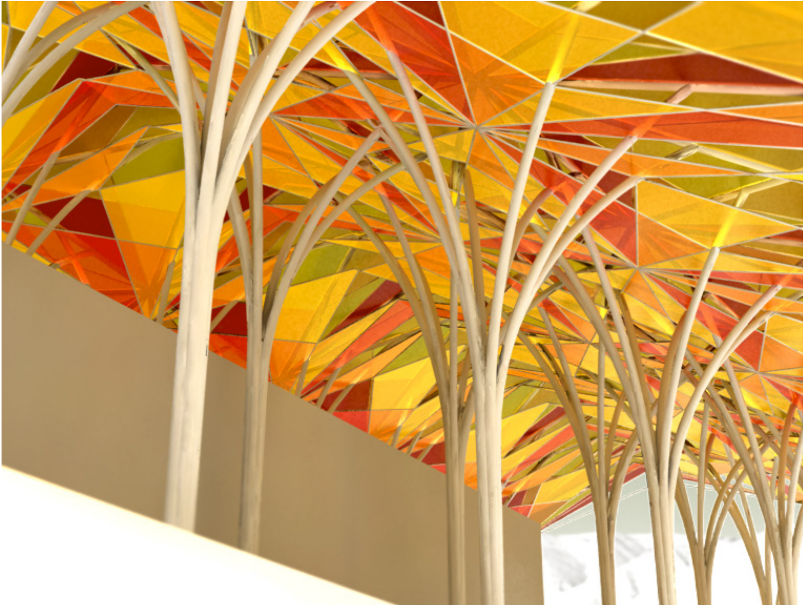
FIGURE120 - GROUND LEVEL VIEW OF PLATFORM STRUCTURE (NO GLAZING)
