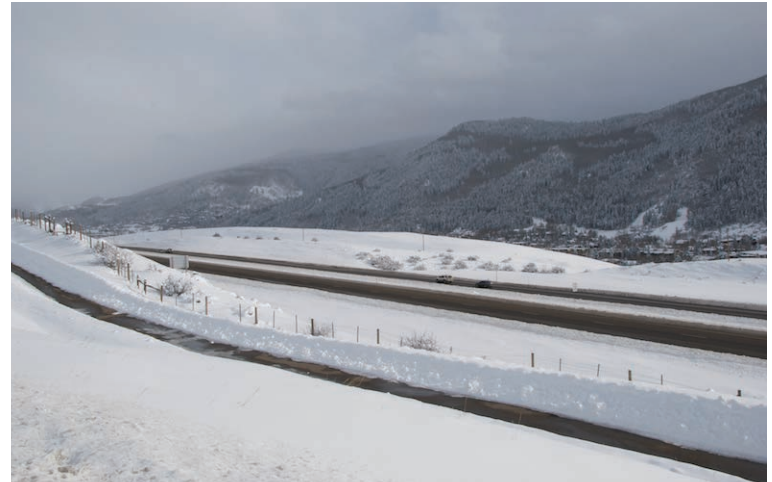
8 - VIEW OF SITE FROM NORTH SIDE OF INTERSTATE 70
